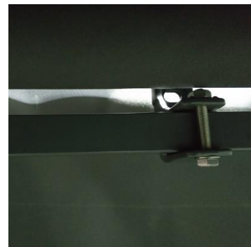
Bolt and nut on wall base bracket
